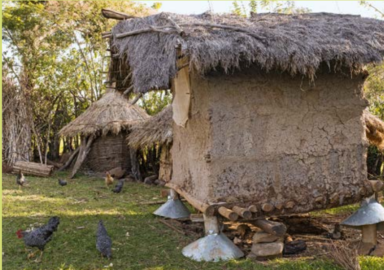
Accessible to neither rain nor rats: the grain safely stored in these improved grain bins.
