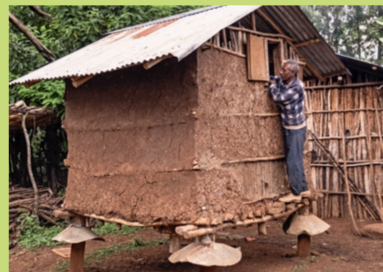
Abera's new grain bin: here the grain stays dry and is secure from gnawing animals
