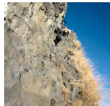
The path used to be highly dangerous.
