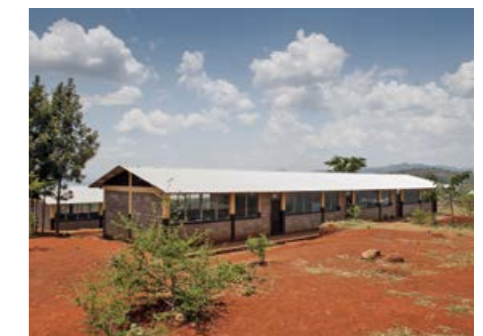
Once a gloomy wooden shack and now a solid building to protect children from the weather and sand fleas: school at Sephera in the Borecha project region.
